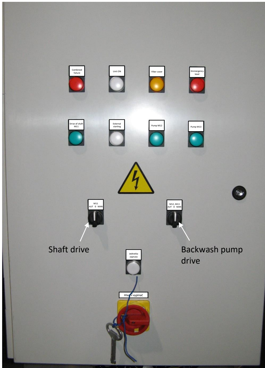
Fig. 41 Switchboard (without sludge pump)
