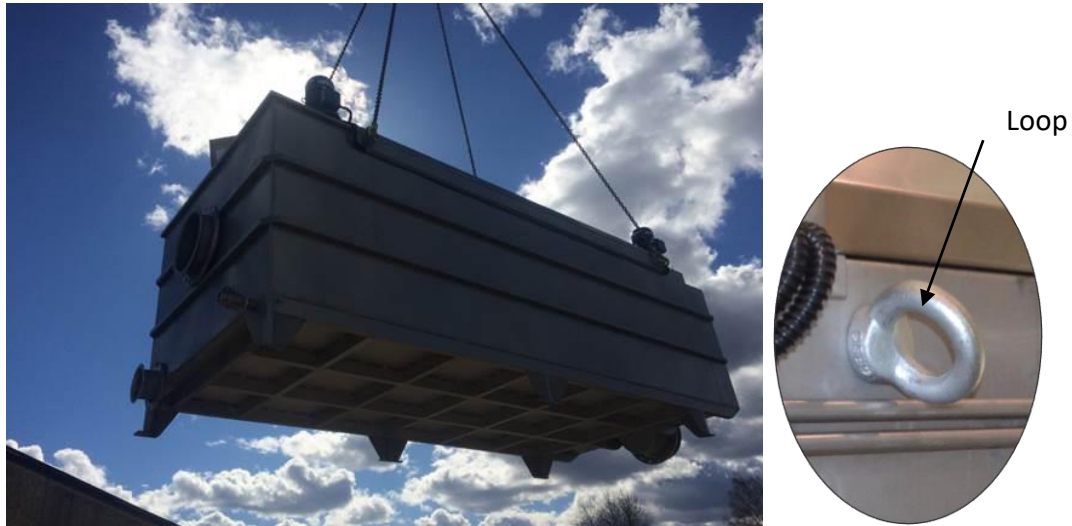
Fig. 27 Filter suspended on ropes, detail
