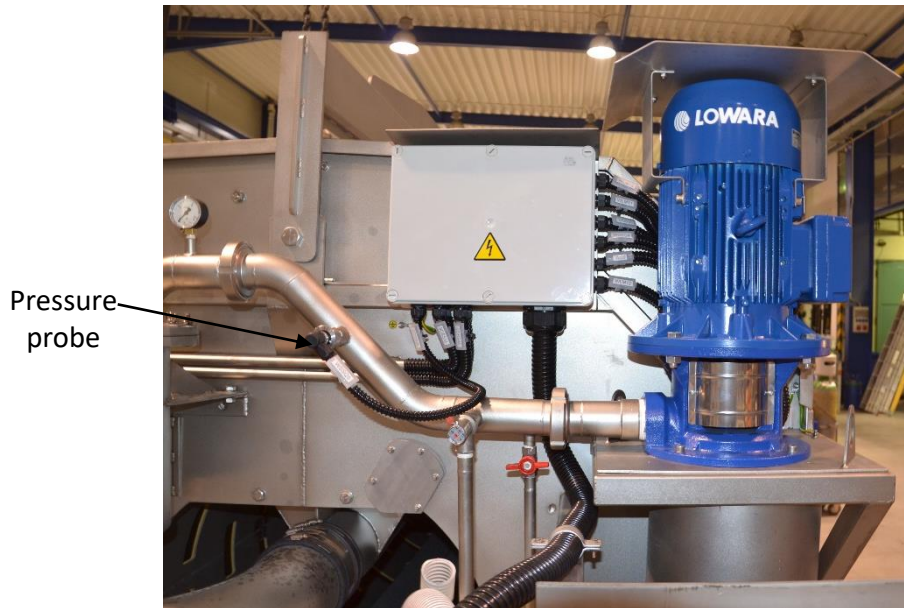
Fig. 11 Probes to check pressure difference
