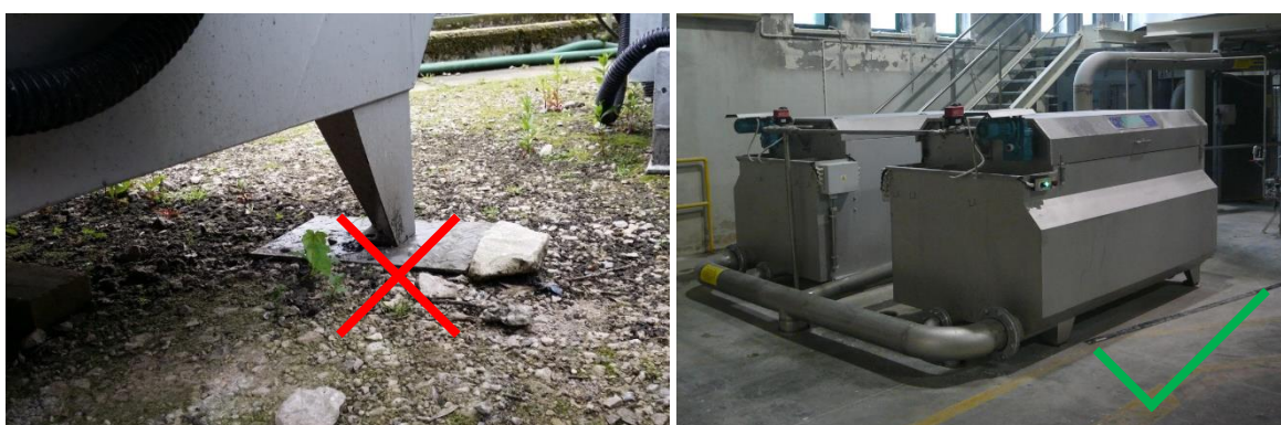
Fig. 33 Wrong and right filter installation
