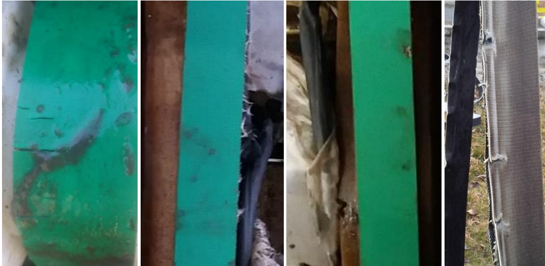
Fig. 50 Damaged drive belt
