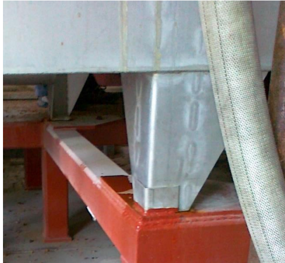
Fig. 38 Back stop around the foot of the filter
